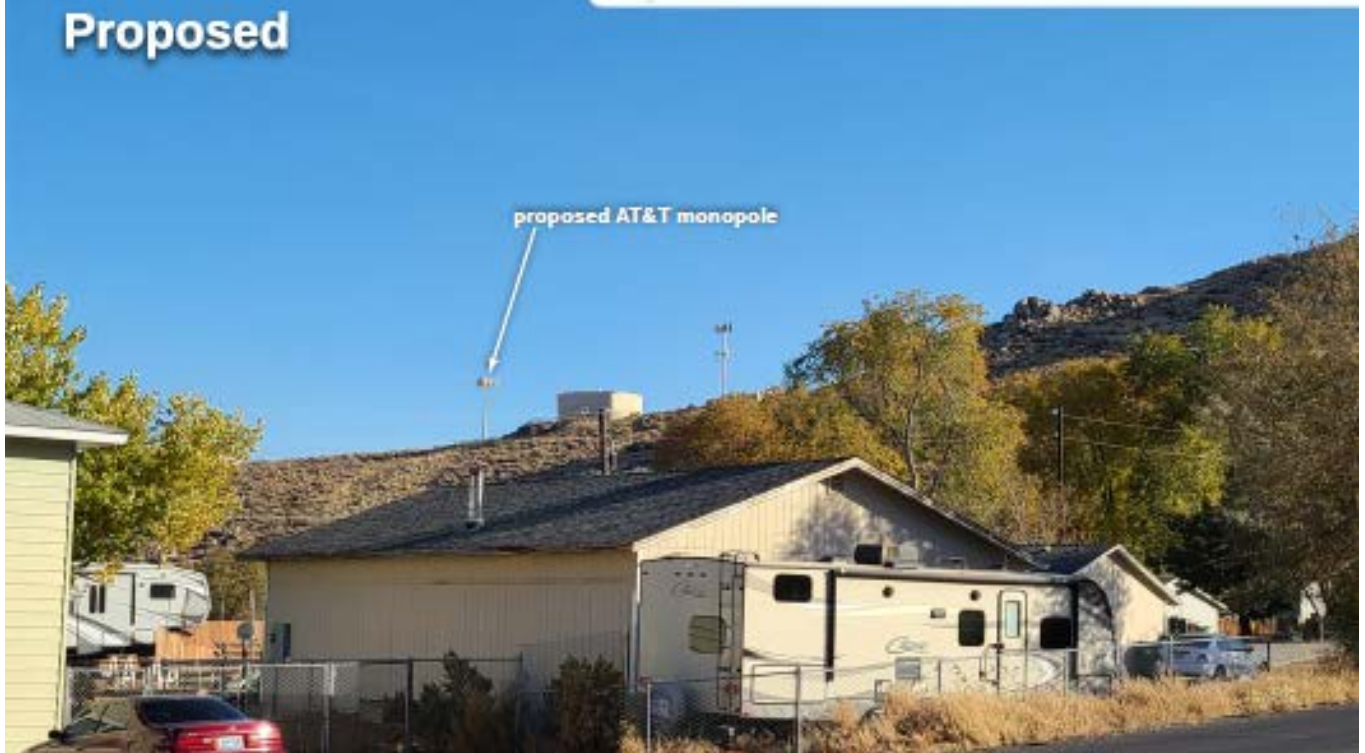
View 4- Looking northeast from Surge Way at Artesian Way
